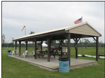
New concrete floor at Nike Field.
